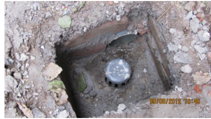
Connecting Recharge Pit
