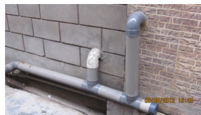
Houses' Pipe Line 1
