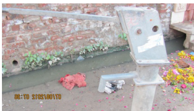
Failed Hand Pump
