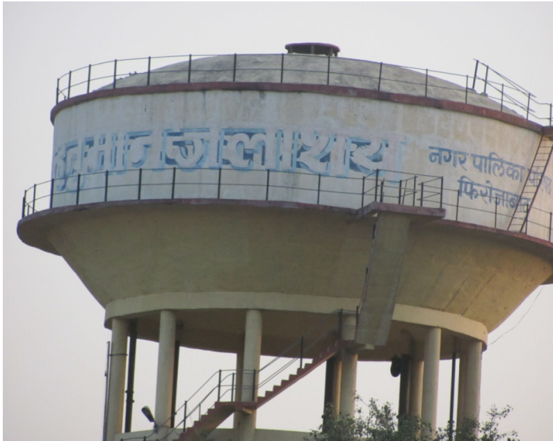
Figure 2: The OH Tank
