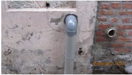
House Pipe Line 2
