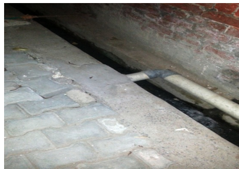
House's Roof Pipe Line Connecting Failed Hand Pump that turned into recharge Pit
