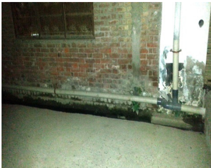
House's Roof Pipe Line Connecting Failed Hand Pump that turned into recharge Pit
